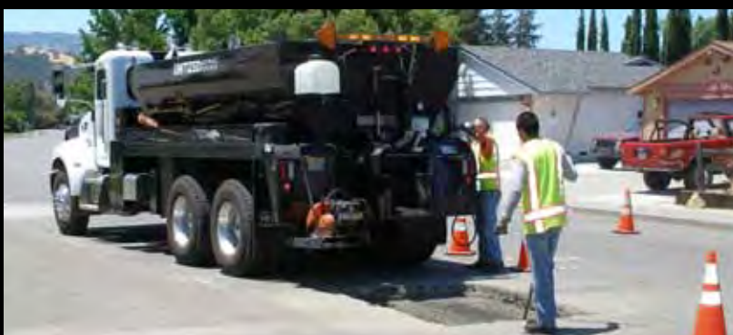
Remove old material, create a firm base and tack the hole edges.
